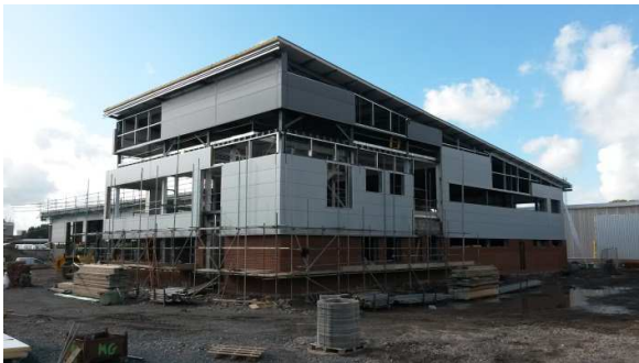
New Worcester Fire station under construction
