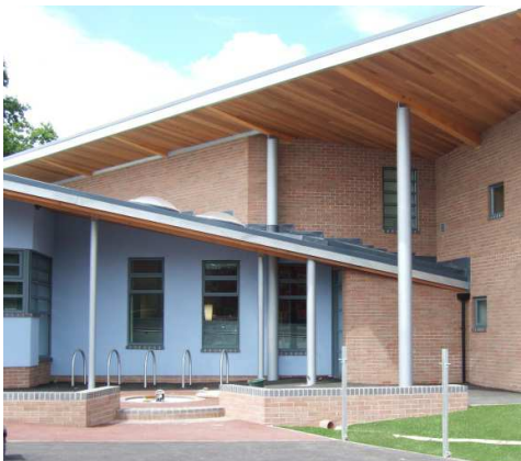
Warndon Community Centre, Worcester, Worcestershire
